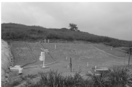
图1 边坡I现场实物图 Fig. 1 Slope I in the field
