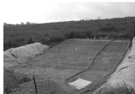
图3 边坡II现场实物图 Fig. 3 Slope II in the field
