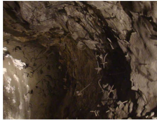
图 7 锚杆加固后围岩破坏现象 Fig.7 Instability of surrounding rock after reinforcement of bolts
