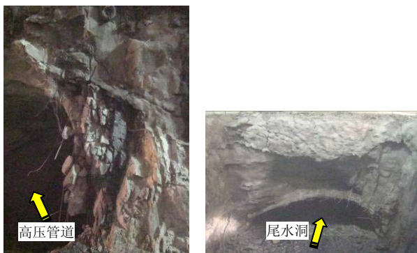
图 20 典型交岔洞口围岩破坏与塌落 Fig.20 Failure and falling of surrounding rock at crotch caverns
