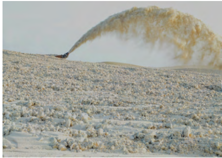
图1 吹填施工 Fig.1 Filling construction
