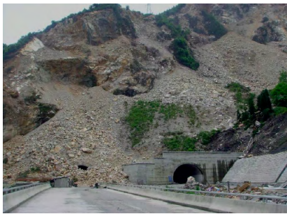
图5 龙洞子隧道出口处边坡崩塌 Fig.5 Slope failure at the exit of Longdongzi tunnel
