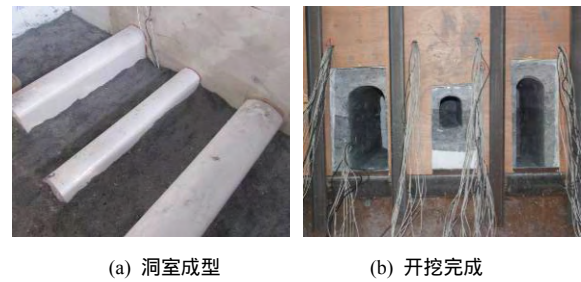
图 12 洞室成型与开挖 Fig.12 Caverns forming and excavation
