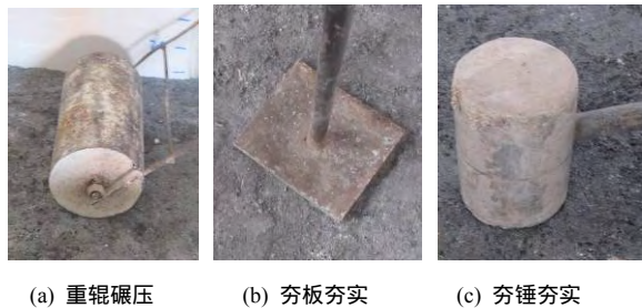
图 10 多手段夯实 Fig.10 Multiple means tamping
