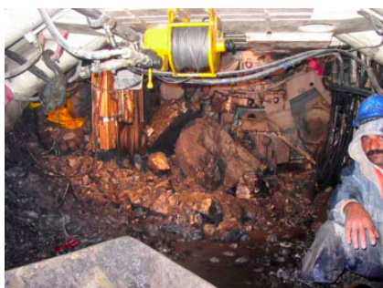
图 1 伊朗 Alborz 隧洞破碎岩体影响 TBM 正常施工 [9] Fig.1 Alborz service tunnel in iran : TBM tunnelling fractured rockmass [9]
