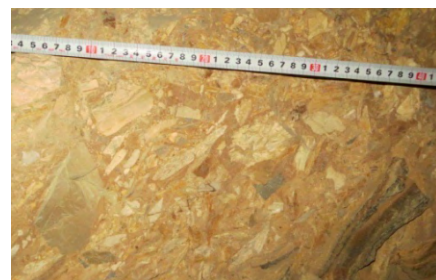
图 3 厂房洞室开挖面揭露的角砾岩 Fig.3 Breccia in the opening face
