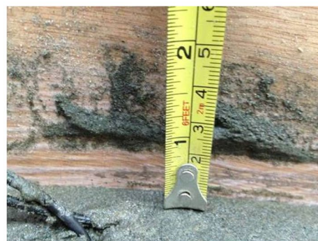
(d) Crest settlement after stopping vibration
