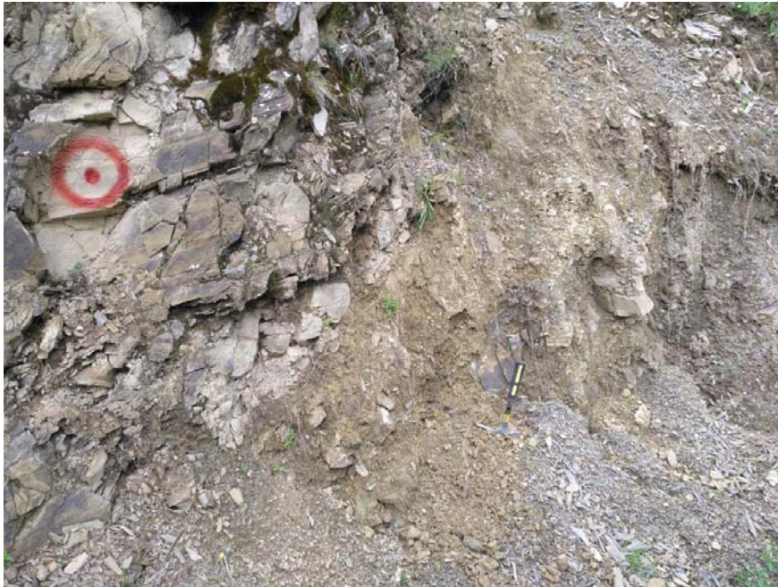
Figure 5 The fault characteristics of Quege ka fault (F27)
