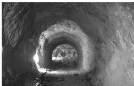
Figure 2 Construction site of experimental branch tunnels B and F .
