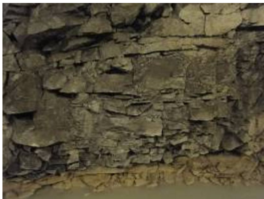
Fig. 11 The platy rock mass on the lower bench of the headrace tunnel #2
