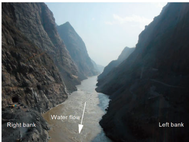
Figure 1. High-mountain valley topography of the Baihetan hydropower plant project site.
