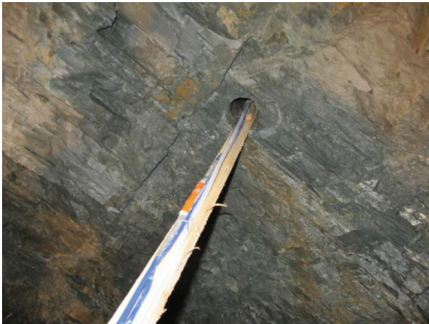
(b) Putting wood sticks into boreholes
